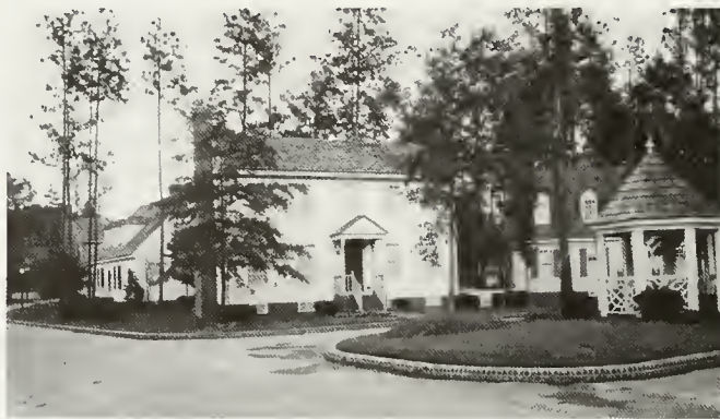
Minimal setbacks and small lots in Cary's Planned Unit Developments (PUDs) are offset by rear service drives and open space areas.
