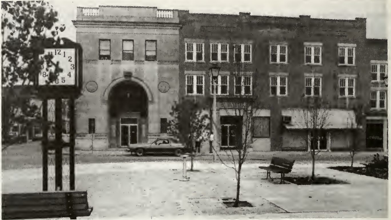
The town government of Ahoskie, North Carolina (population 5,000), donated this 20,000 square-foot downtown building for conversion into a small business incubator.
