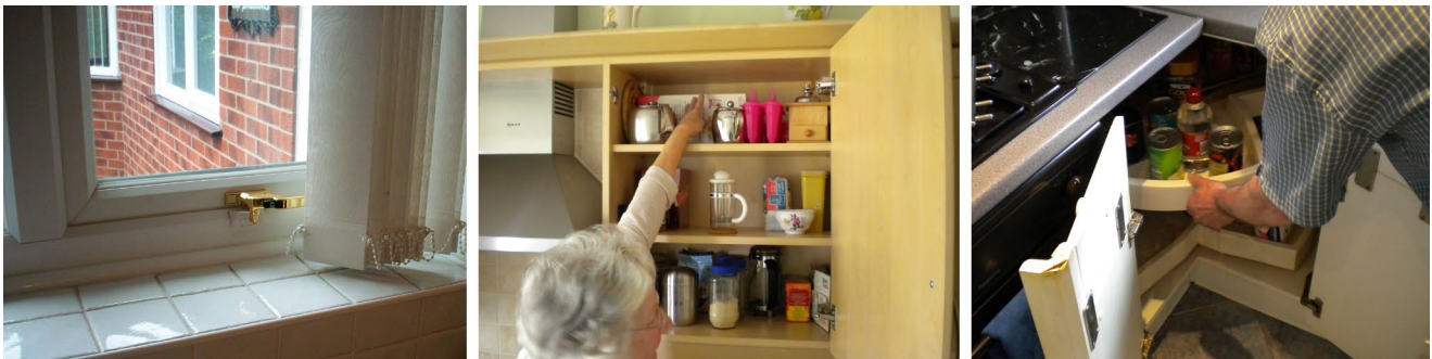
Figure 4. Reaching and stretching: (1) Handle at bottom of window making it easier to reach, (2) Cupboards located at a more convenient height, (3) Carousel shelf providing easier access.
