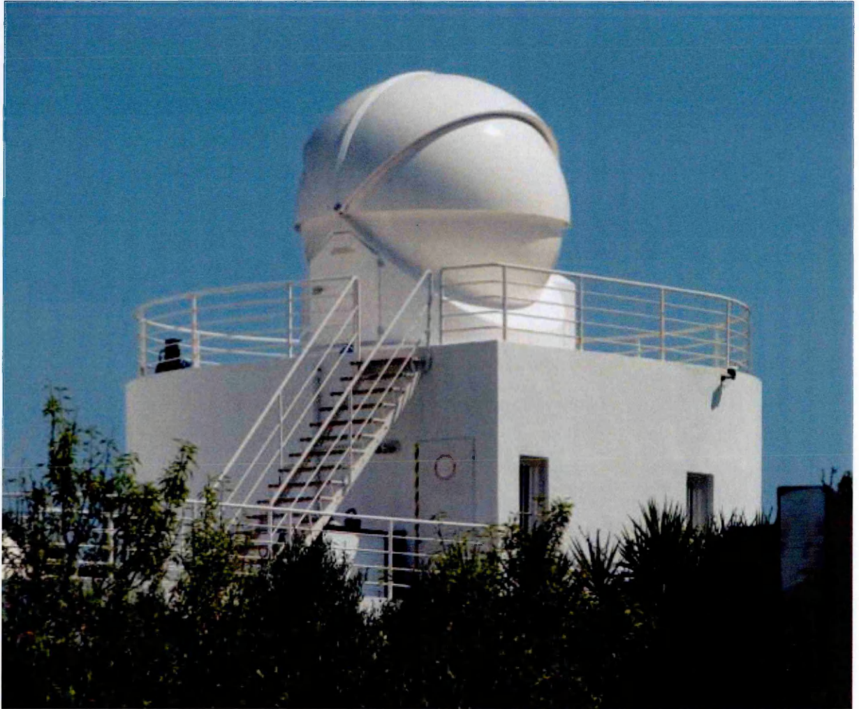
Figure 2.2: PIRATE's new dome enclosure, the Baader Planetarium All-Sky 3.5m dome.
