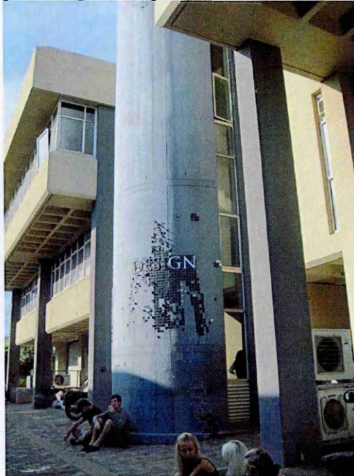
Image 13: Design building entrance - Central campus
