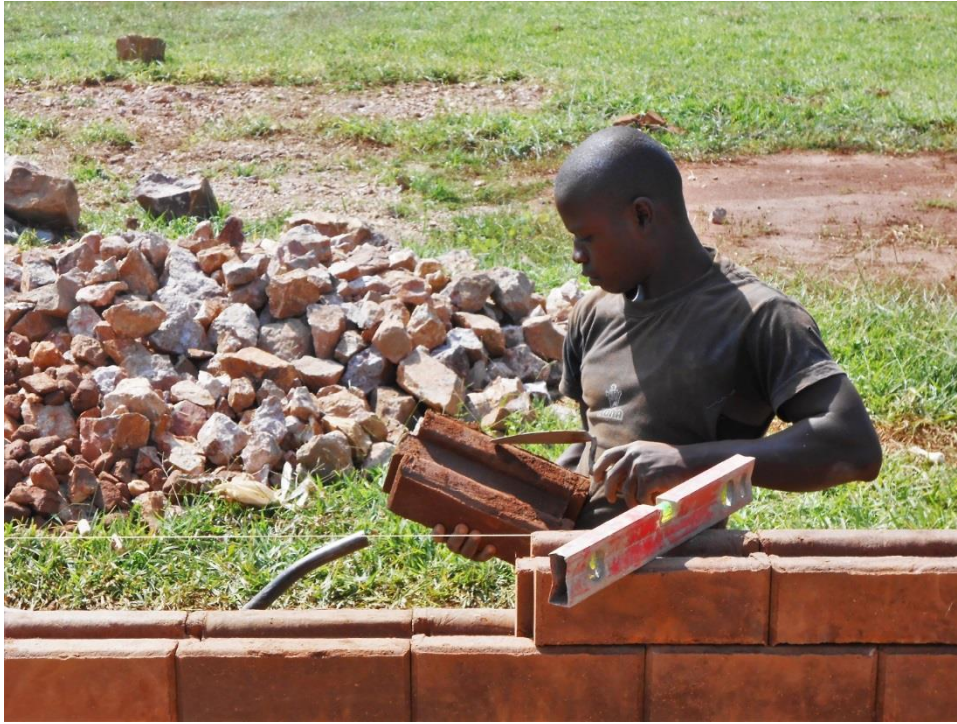
Figure 1-5: An example of cement-stabilised soil construction using interlocking stabilised soil blocks (ISSB). Image courtesy of Haileybury Youth Trust.
