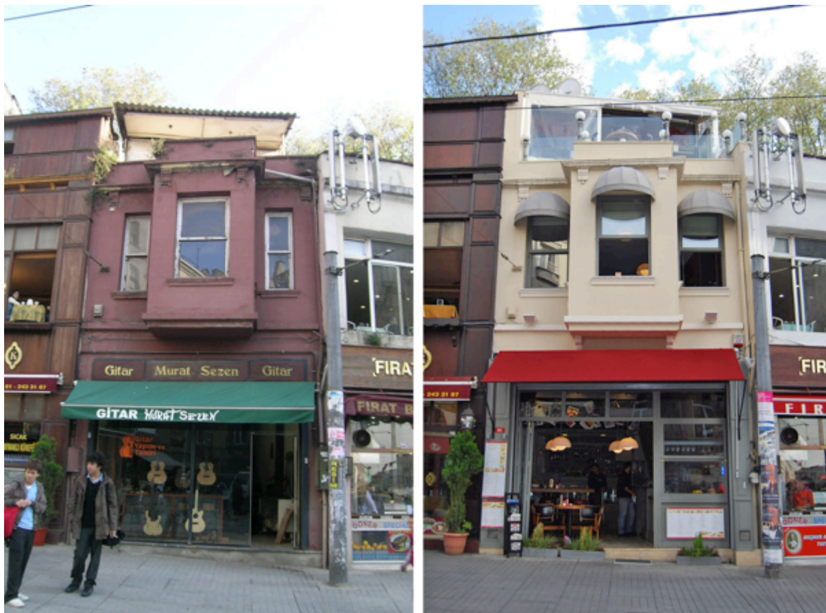
Figure 4-3 A restaurant replaces a guitar shop, expanded to the rooftop and changed the façade Source: Planning Department at Beyoğlu Municipality
