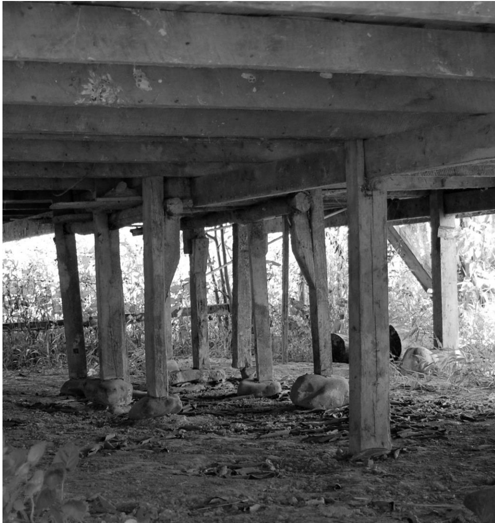
Figure 2a: Local hardwood structures mounted on plinths of large stones form the nearby riverbank. Underside of the Pa'Dalih longhouse constructed in the late 1970s.
