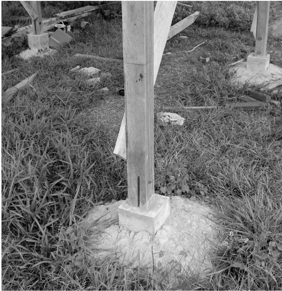
Figure 2c: Concrete footing with metal mounting plate. Close up of the foundations of the house in Figure 3.
