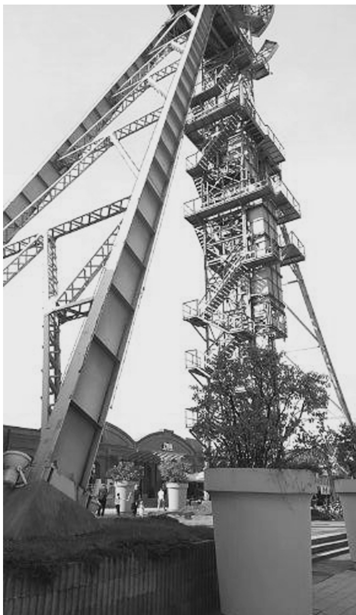
Photo 11. Silesia City Center erected on the site of the former Gottwald coalmine, Katowice 2017 (A. Kuncce)
