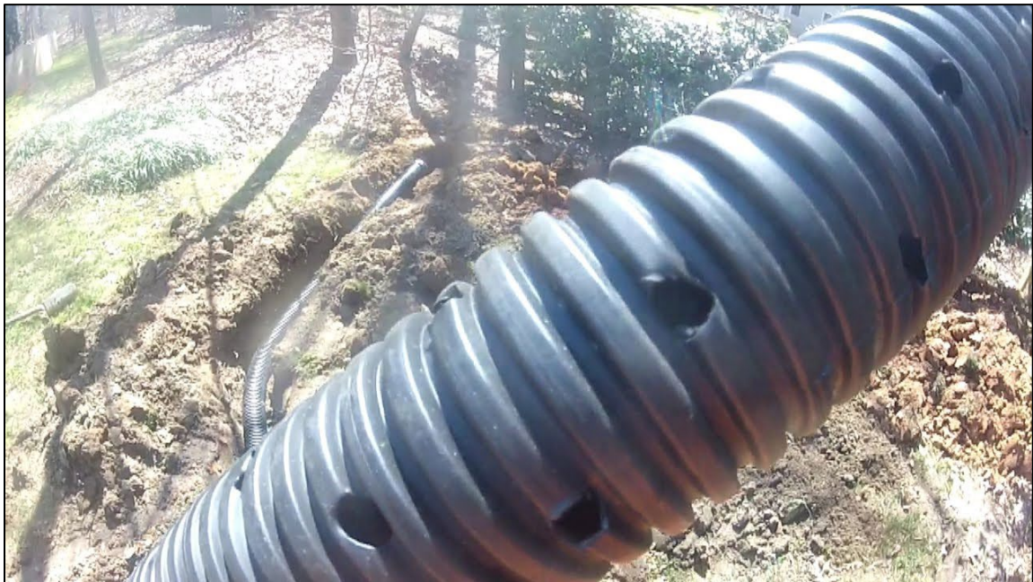
Figure 6. An Example of a Perforated Pipe Used in a Septic Drain Field.
