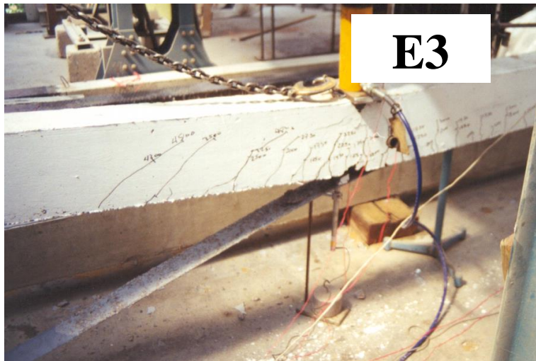
Figure 5 Plate separation of CFRP laminates at soffit mid span (beam E3)
