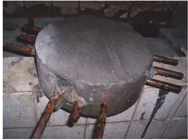
(b) Reinforced concrete blocks
