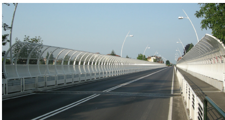
FIGURE 2: Deck of “Ponte degli Alpini.”
