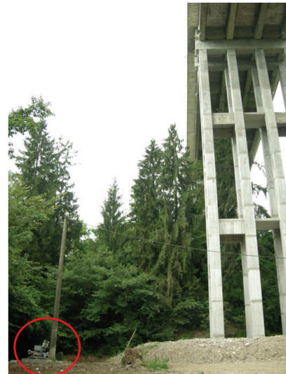
FIGURE 13: The radar (red circle) placed on a basement under the span.
