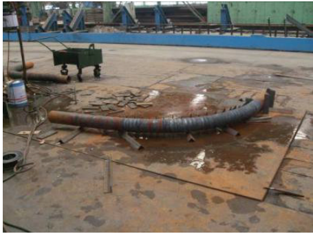
FIGURE 4: Manufacturing procedure of steel tube in factory.
