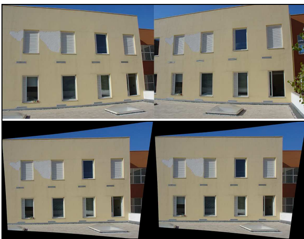
Figure 7. Rectified and rotated left image of the above pair (image axes convergence of 32°).
