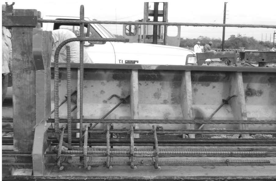
Fig. 4 Picture of end zone reinforcement.
