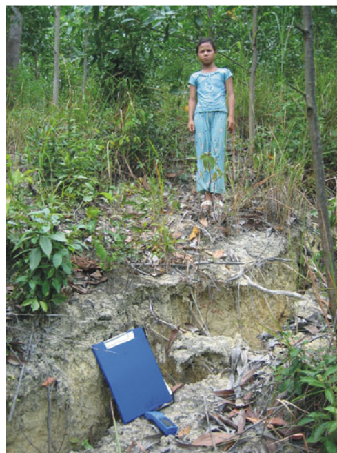
Fig. 13 Signs of potential landslides in Van Canh district (tension crack and scarp at the top)
