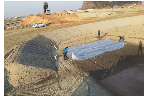
FIGURE 13: Plastic film application for the field test.
