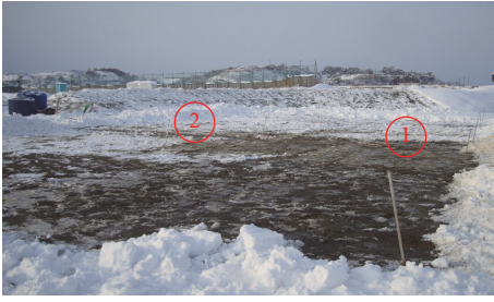
FIGURE 14: View of the field test site on the 21st day of test.
