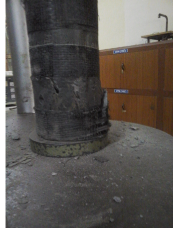
FIGURE 5: Failure pattern of NC-20-2.
