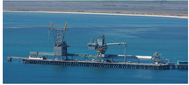
FIGURE 8: Parallel operation of old (left) and new (right) ship unloaders on the Tiwai wharf. (Photograph by K Lawry.)
