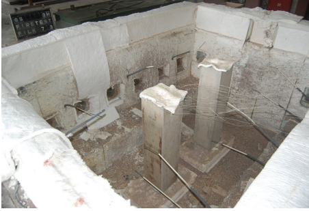
FIGURE 3: RC columns in furnace before fire test.
