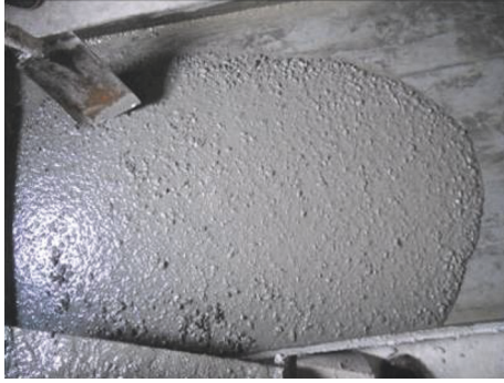
FIGURE 2: Status of the concrete mixture.
