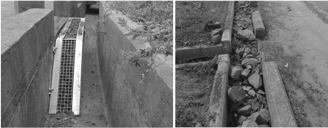
Fig. 5 The artificial corridor installed in the EIL ( left ) and covered with aggregates
