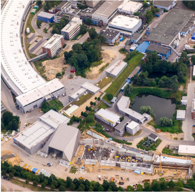
Figure 11. Aerial view of the FLASH Facility at DESY, Hamburg. The accelerator is from top right to the lower left, with the two experimental halls; Kai Siegbahn hall (left) and Albert Einstein hall (right) in the lower left corner. The curved hall (left) and the construction site (bottom) belong to the synchrotron radiation facility PETRA III. Courtesy: DESY, July 2014.
