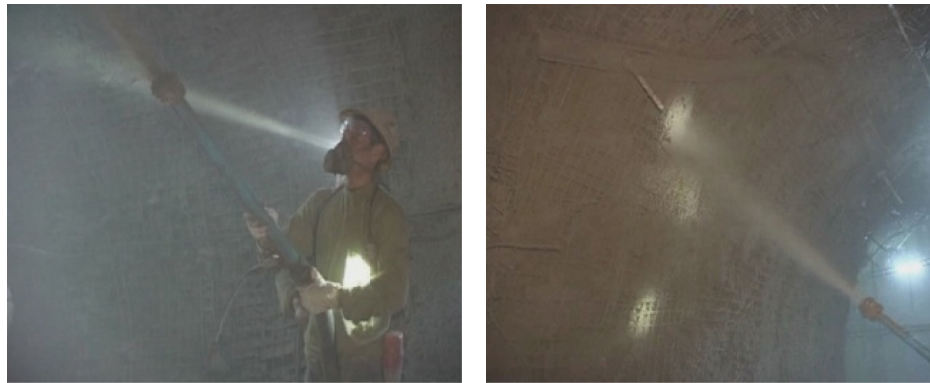
FIGURE 8: The site of wet spraying.
