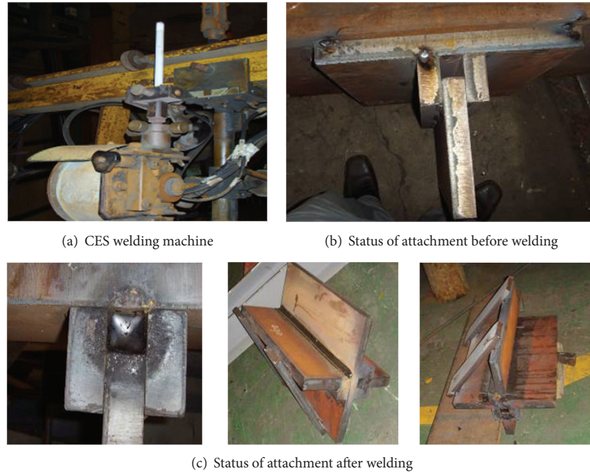
FIGURE 4: ESW welding status.
