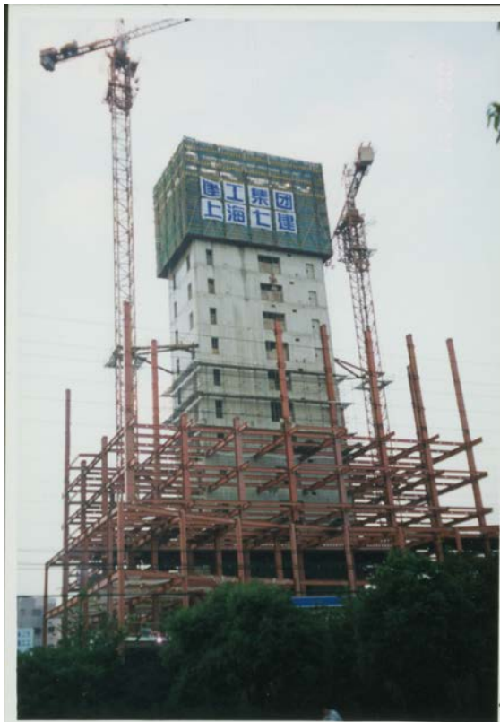
Fig. 13 The prototype building under construction (a) concrete tube nearly completed; and (b) composite structure nearly completed
