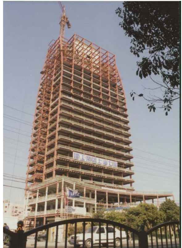
Fig. 13 The prototype building under construction (a) concrete tube nearly completed; and (b) composite structure nearly completed
