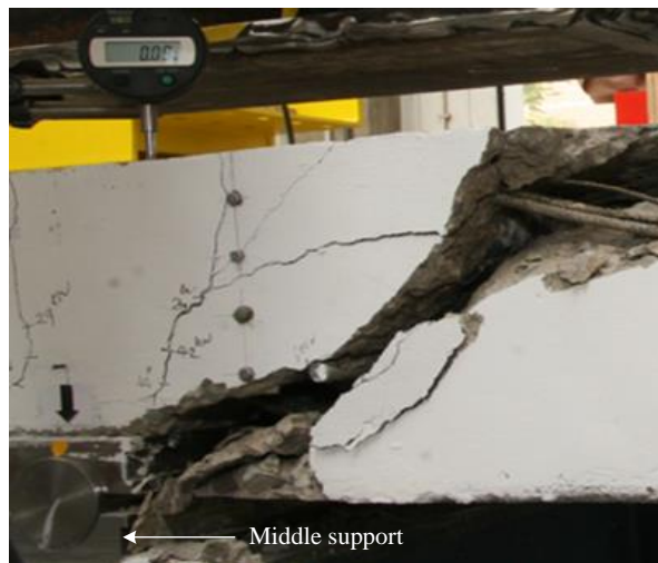
Figure 3–11: Compressive flexural-shear failure at middle support of slab C–B–OO
