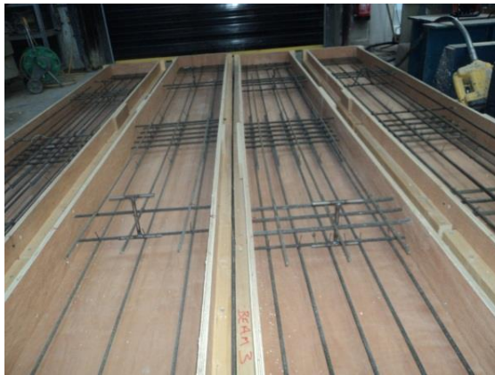
a) Reinforcement cages in forms
