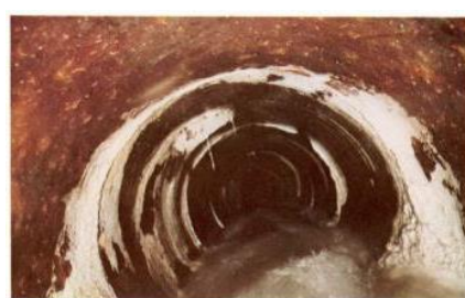
(6) Slight joint displacement, heavy encrustation, lightly slimed, clayware pipe, 450mm diameter, k_s^r = 6\text{mm} .
