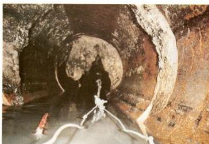
(15) Severe encrustation, major debris on invert, clayware pipe, 305mm diameter, k_s^r = 30\text{mm} .
