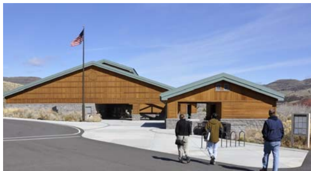
Figure 9: The Thomas CONDON Visitor's Center at John Day Fossil Beds National Monument in Oregon, USA (URL: http://www.nps.gov/joda/ ), contains a gift shop, museum, preparation laboratory visible to visitors through glass windows, and research collections, library and space for researchers. The Monument is visited by tourists and scientists alike interested in seeing the Eocene to Miocene formations and fossils exposed in three different areas of east central Oregon.
