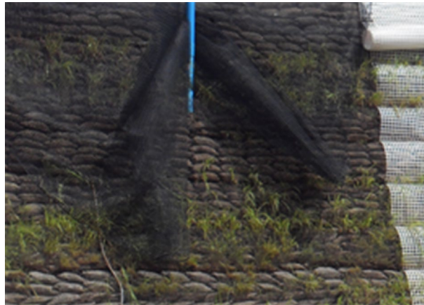
Fig. 6 The soil bag facing to retain backfill material
