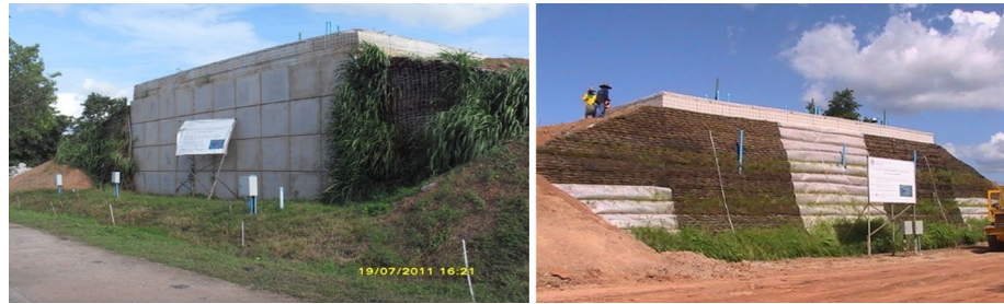
Fig. 9 Photograph showing vertical face and sloping face showing metallic and polymeric reinforcements respectively
