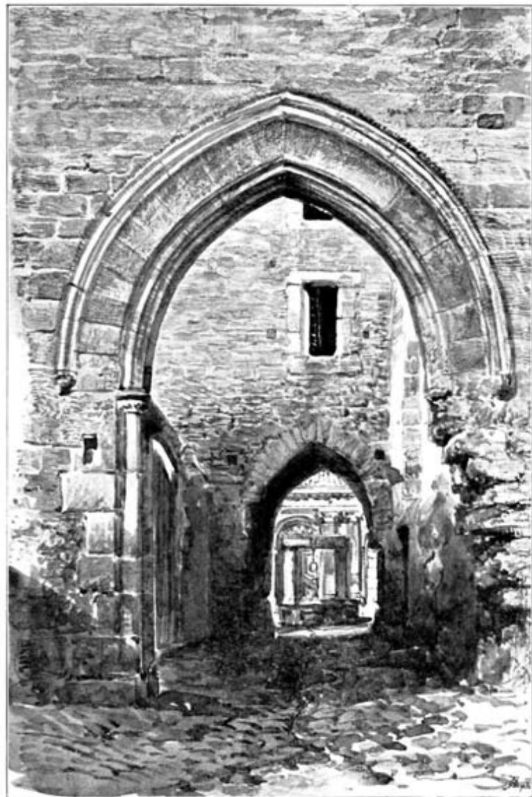
RUINS OF MONASTERY, VILLENEUVE.
