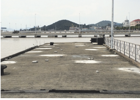
FIGURE 1: The cores drilling site.
