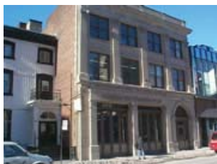
Photo 2.1 : Station CV (RSQA)
