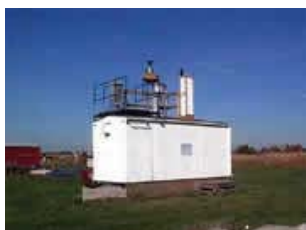
Photo 2.3 : Station Ouest (RSQA)
