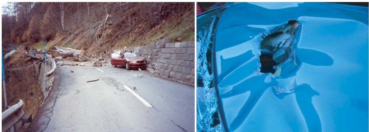
Fig. A1.13 In mountainous areas, transportation corridors are regularly subject to rockfall activity: (a) In November 2003, rockfall obstructed the cantonal road connecting Stalden with Saas-Almagell (Eisten, Valais Alps); (b) On May 1, 2003, a small rock ( \varnothing 30 cm) crashed through the roof of a car passing the Stägjitschuggen rock cliff near St. Niklaus (Valais Alps), killing the passenger (20min 2003). (Photo courtesy by Kantonspolizei Wallis [a, b], used with permission)
