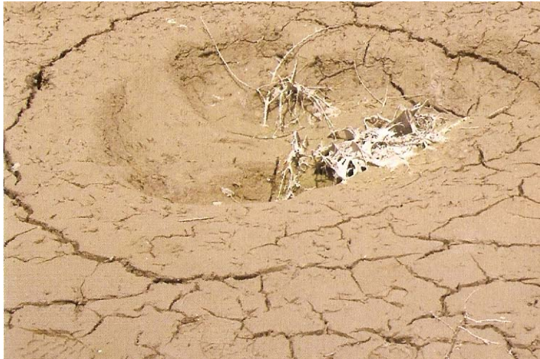
Figure 4. A sinkhole in reservoir area about 40 m from the dam heel.
