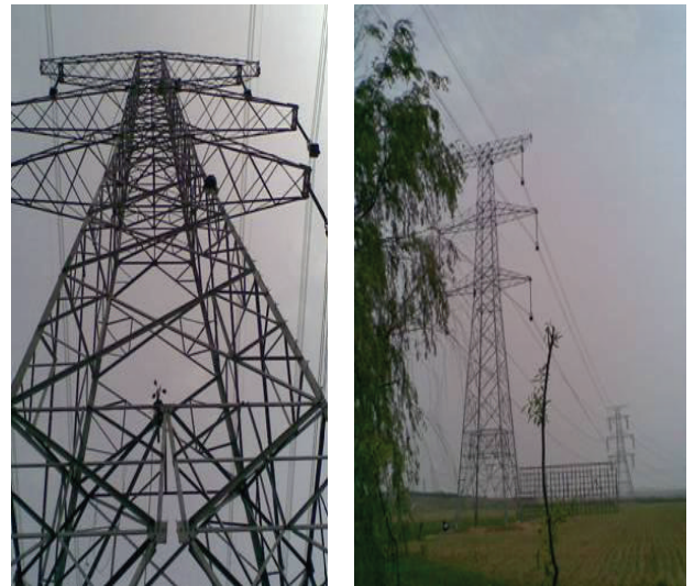
FIGURE 4: SZ21-type tangent transmission tower in Liaoning province.
