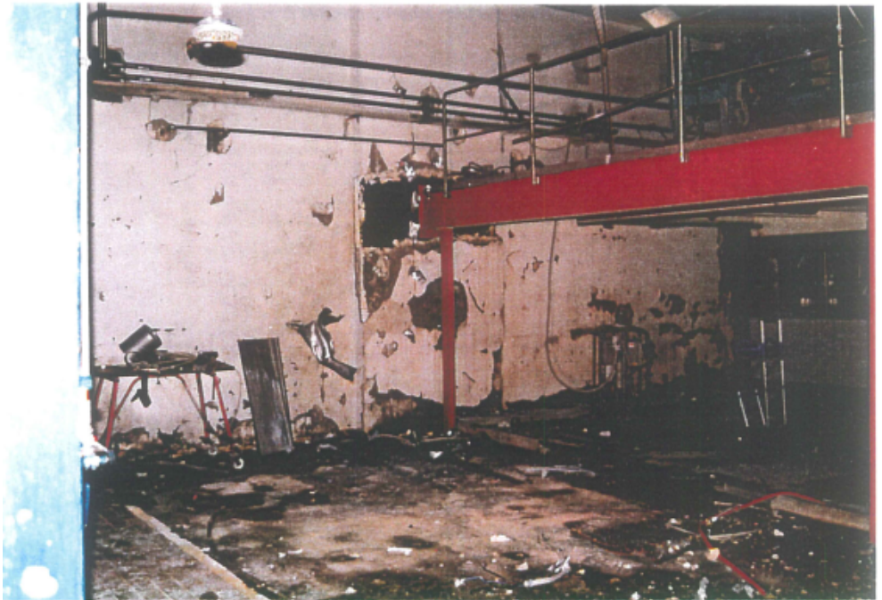
Figure 3 Tank fragments lodged in heavy concrete wall (marked as location b in Figure 1). Photo courtesy of company.
