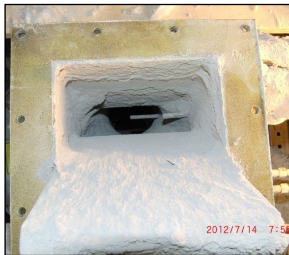
Figure 95 – Top view of the interior of the bottom stage after the PoC experiments. Two thermocouples are visible: Particle outlet #2 and inlet to bottom stage.
