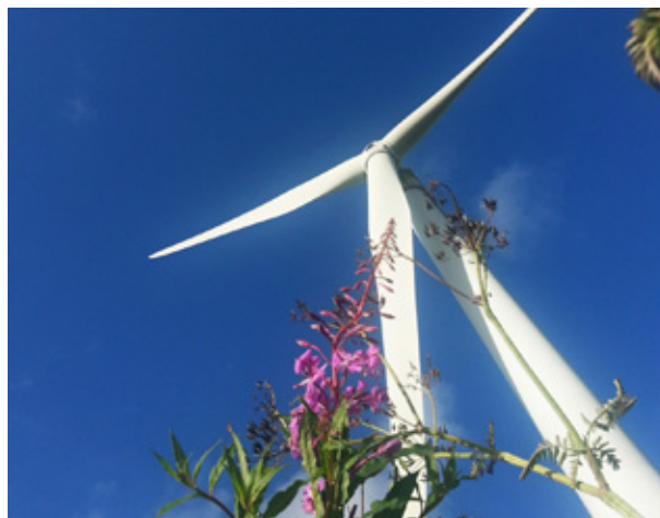
Fig. 3. The NM80 2.3 MW test turbine at Tjæreborg Enge (Courtesy Dong Energy)
