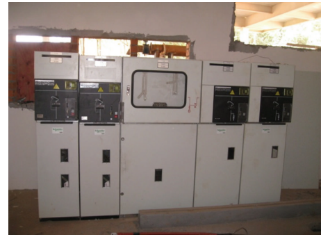
FIGURE 5: The solar controller of solar photovoltaic systems in West Lushan highway service area.
