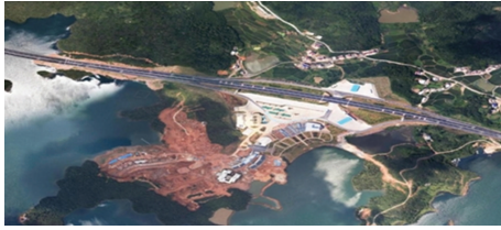
FIGURE 1: The aerial view of Lushan highway service area.
