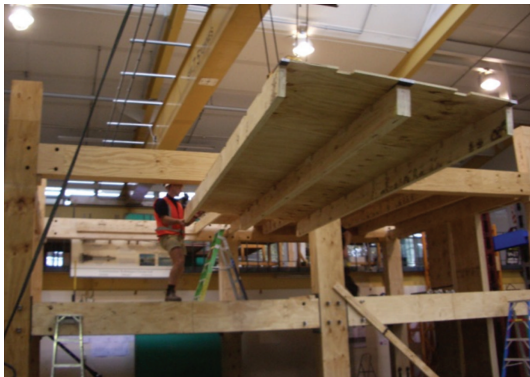
FIGURE 4: On-site assembly of floor unit in laboratory.
