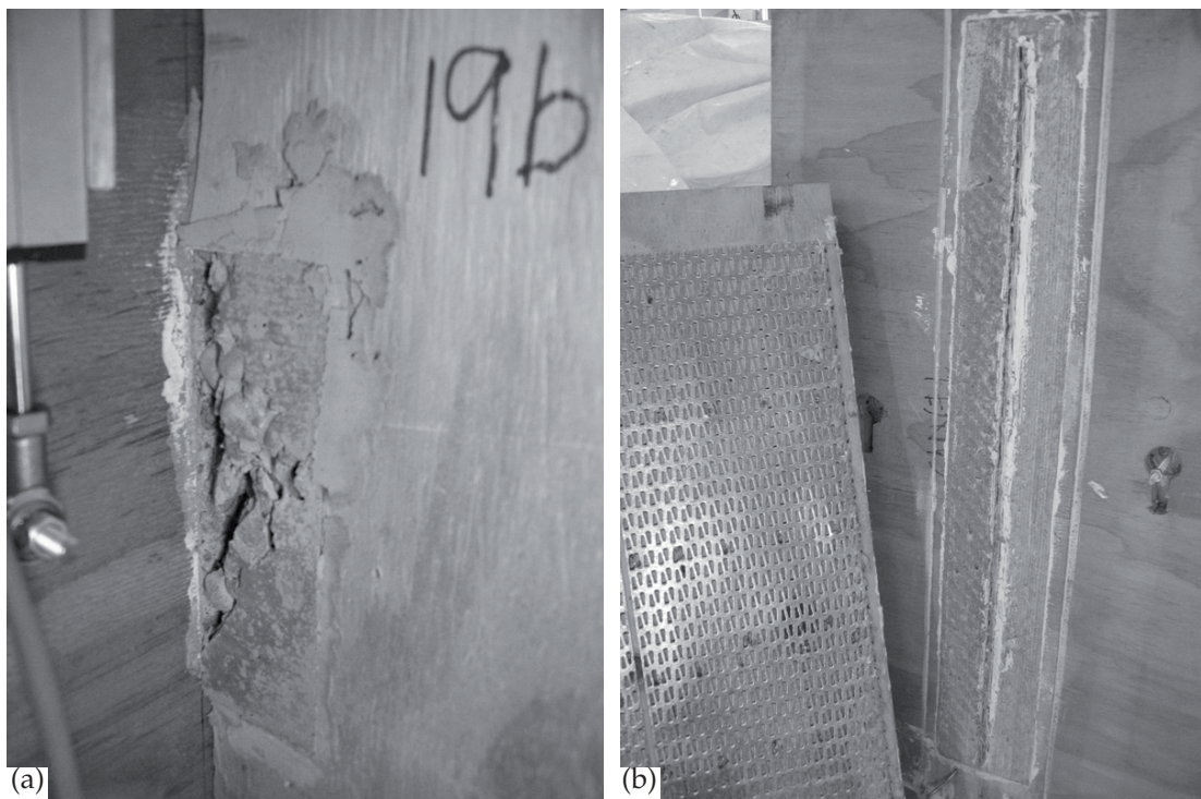
Figure 9: (a) Rectangular notched connection failure – shear in concrete length, and (b) toothed metal plate connection failure – plate tearing along length of plate.
