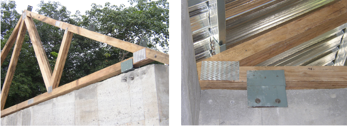
Fig. 1 Rubberwood LVL trusses for a research station
