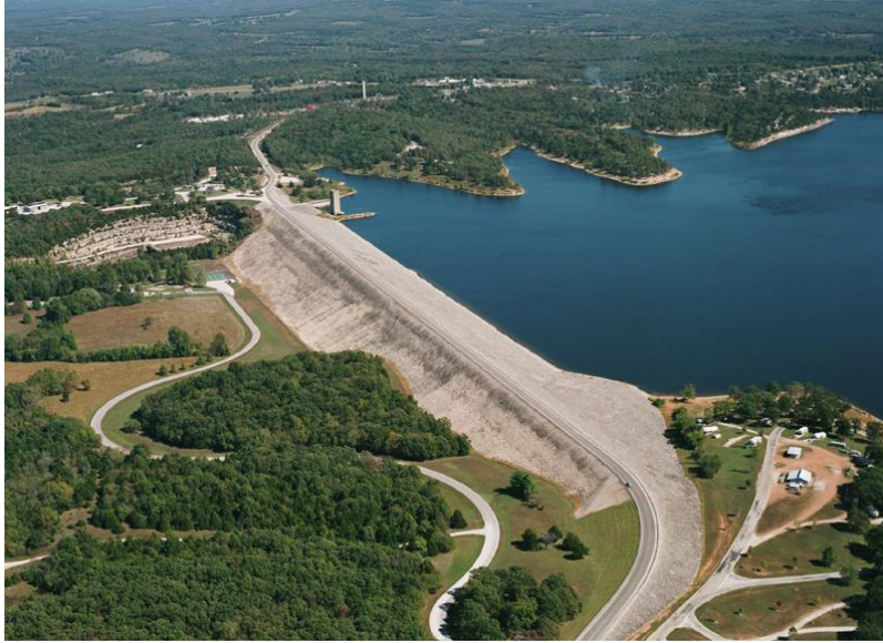
Figure 40 Image of an Earth Dam (U.S. Army Corps of Engineers 2013).
