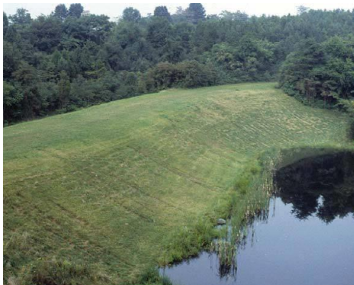
Figure 23 Image of a Reservoir Embankment (VirginiaTech 2007).
