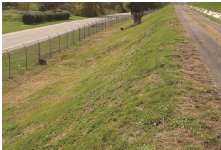
Figure 7 Image of a Road Embankment (Terracon 2013)
