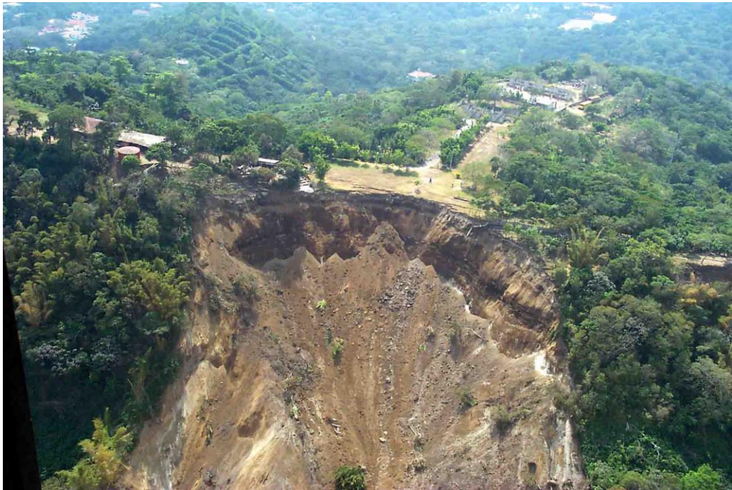
Figure 3 Image of the Las Colinas Landslide (U.S. Geology Survey 2010).
