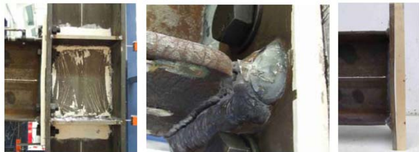
Figure 2.21: Column web panel, beam flange failure and end-plate deformation for J-3.3
