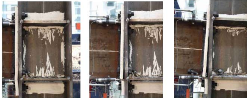
Figure 2.20: Column web panel, end-plate and bolt failure for J-3.2
