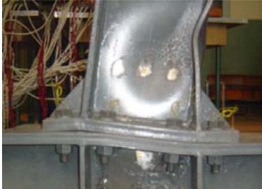
Figure 2.34: Failure mode for EPC-4
