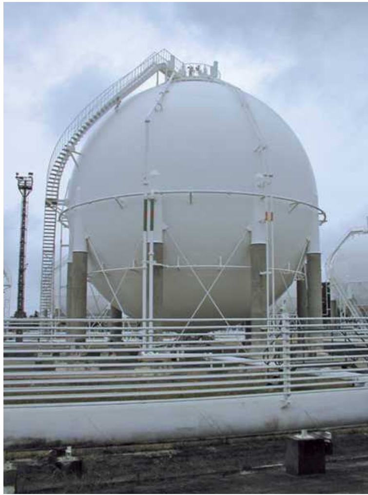
Figure 22.1- Spherical tank methane gas-filled
