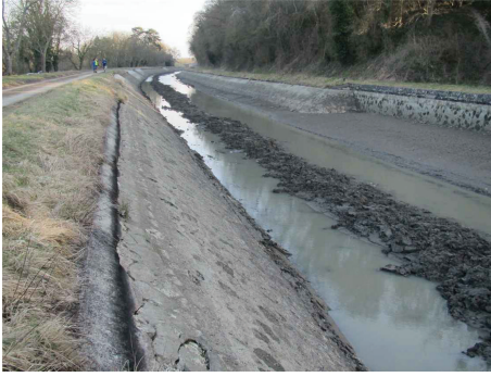
FIGURE 1: General view of the embankment.
