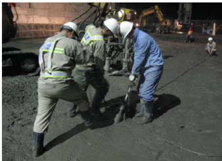
FIGURE 6: The burying process of cable.
