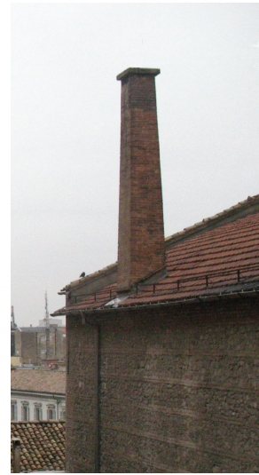
FIGURE 3: An old masonry chimney.
