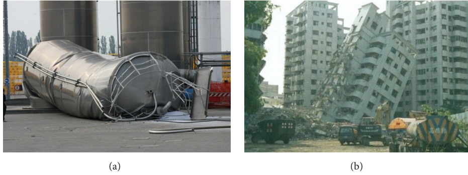
FIGURE 1: Catastrophic collapses due to earthquakes.
